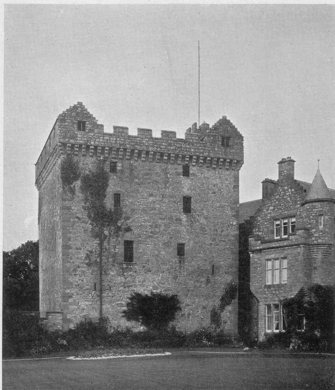
Fig 2. COMLONGON CASTLE: VIEW FROM SOUTH.
