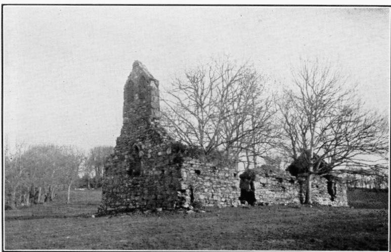
Plate VII.—ST. TRINIAN'S CHURCH, BEFORE RESTORATION, FROM THE SOUTH-WEST.
