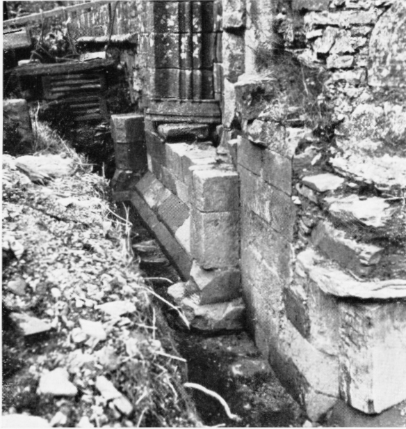
Plate V.—WHITHORN. SOUTH WALL OF NAVE (12th CENTURY)
